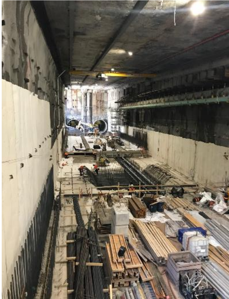
REBAR INSTALLATION
